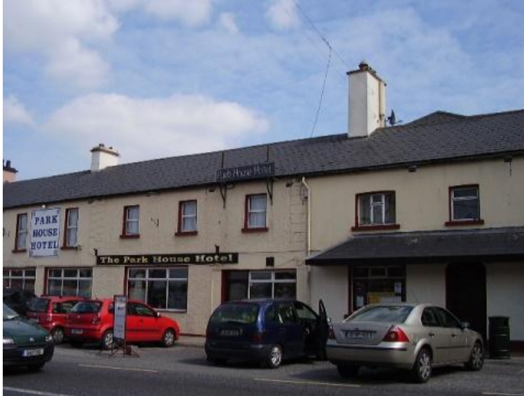
Transmitter Site Photo
